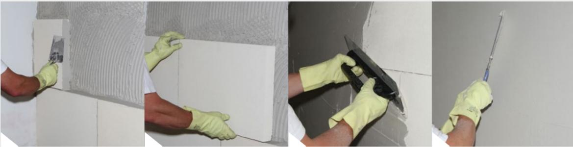
A bead of KÖSTER Hydrosilicate Adhesive SK is applied along edges of the boards to make sure that the joints are fully filled.
